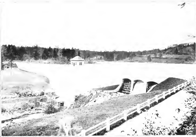
THE WIGWAM DAM AND RESERVOIR OF WATERBURY'S MUNICIPAL WATER SYSTEM
